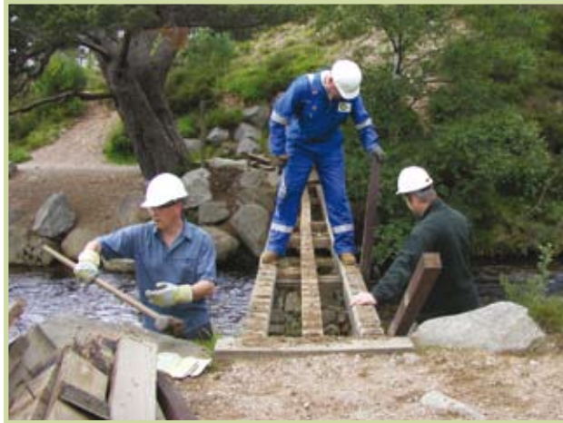
FCS - Bridge building at FCS Glenmore
